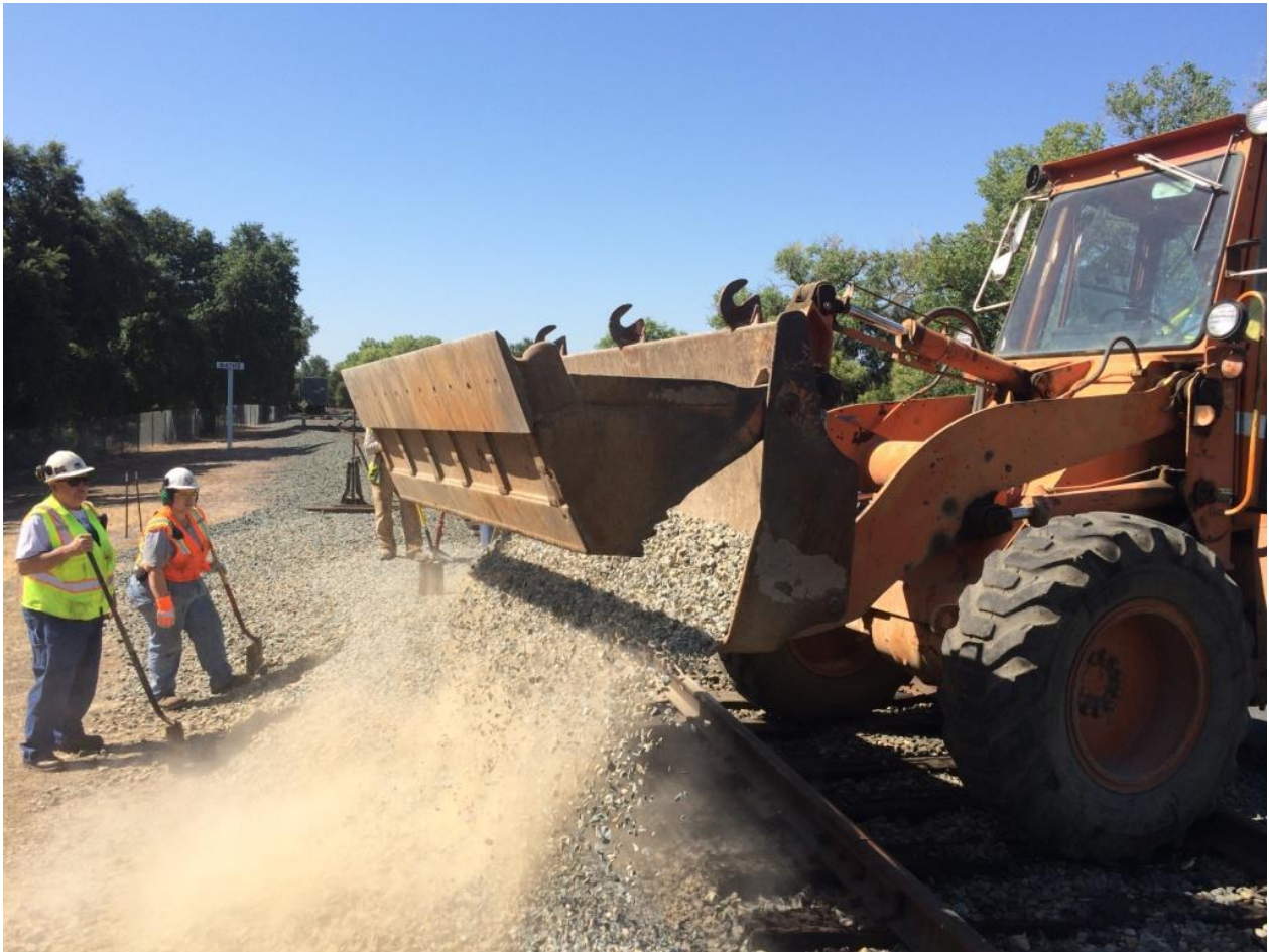
Harry and Heather guide the placement of fine rock near Switch 17
