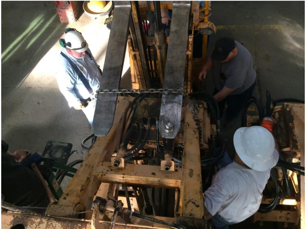
The view from the roof: Frank, Gene, and Mike H., secure the work-head to the forklift for removal from the old-old tamper
