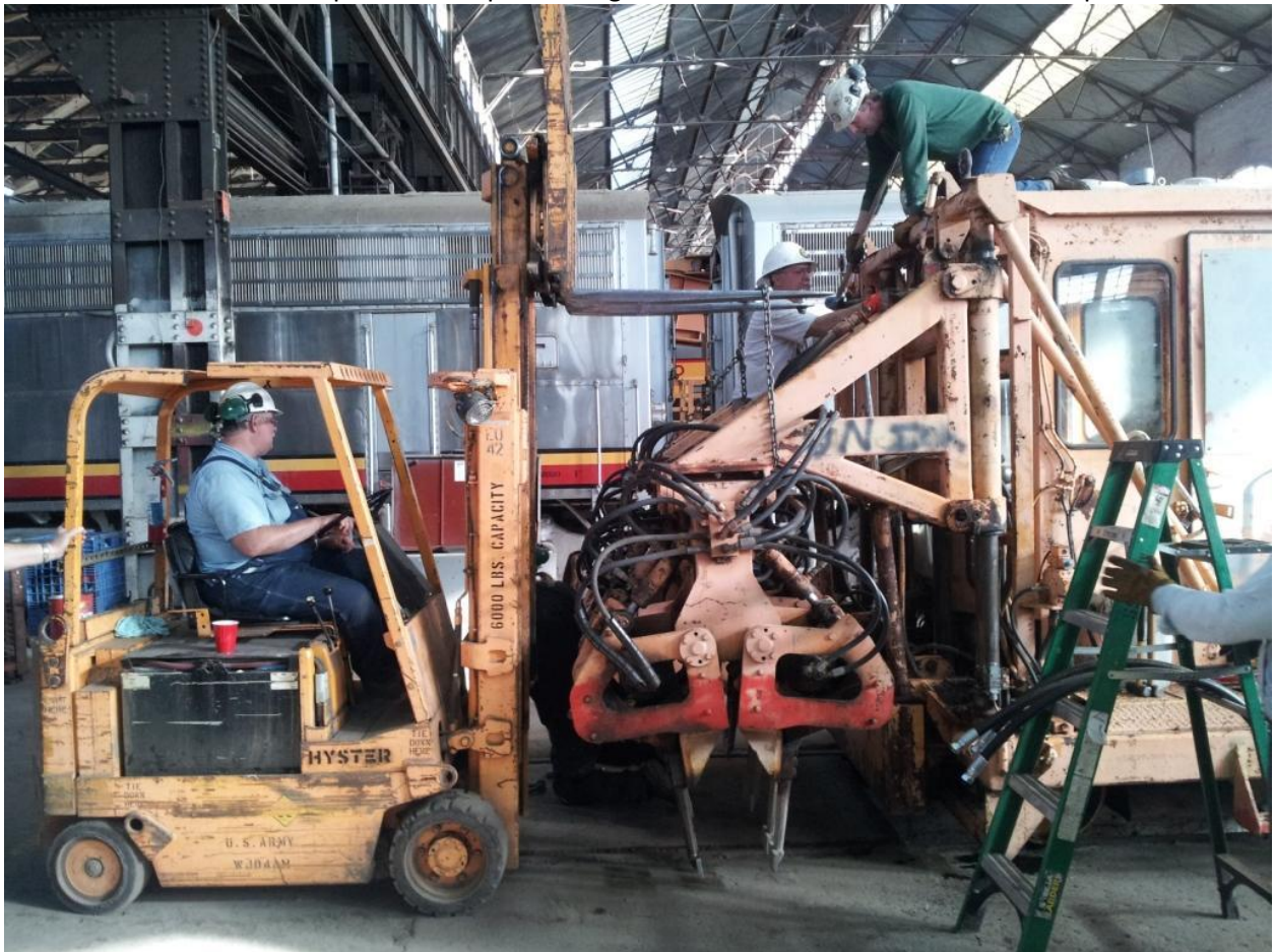
Removing the support pins in tight quarters required a bit of team-work
