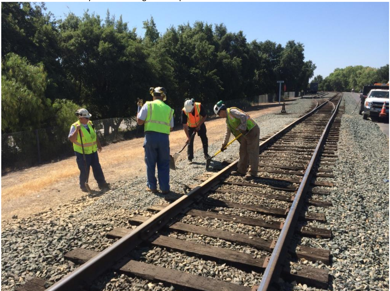
Harry, Clem, Fred, and DJ spread and smooth the new surface
